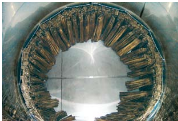
Tank Fans installed in a tank (top view).
